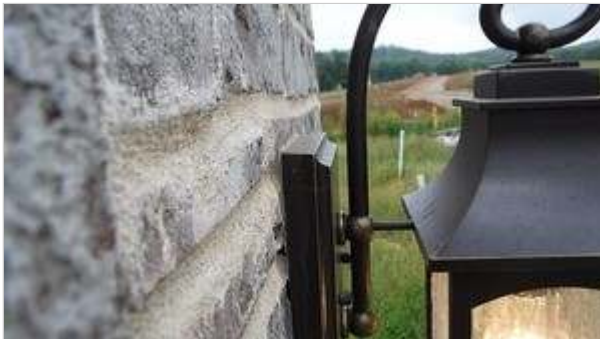
Driveway lights, gapped caulking
