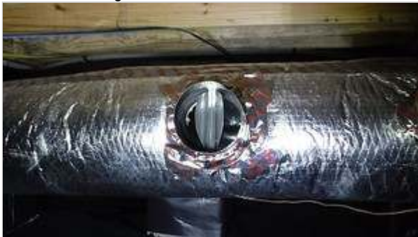
Crawl space positive ventilation system
