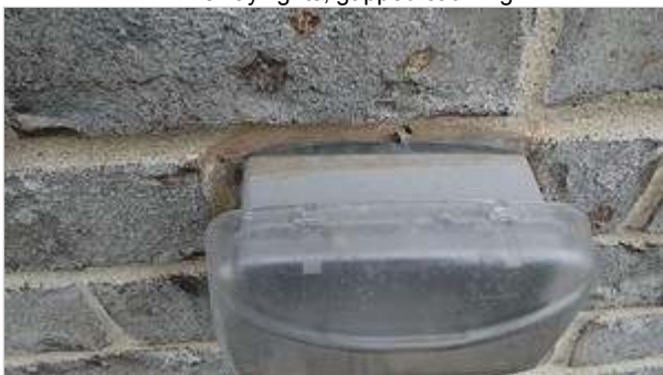
Rear electrical outlet, gapped caulk
