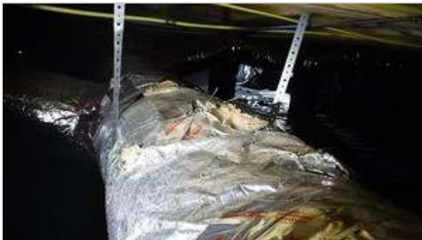
Damaged HVAC insulation under kitchen
