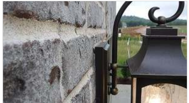
Driveway lights, gapped caulking
