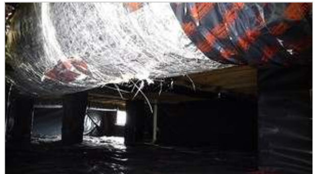
Damaged HVAC insulation under kitchen
